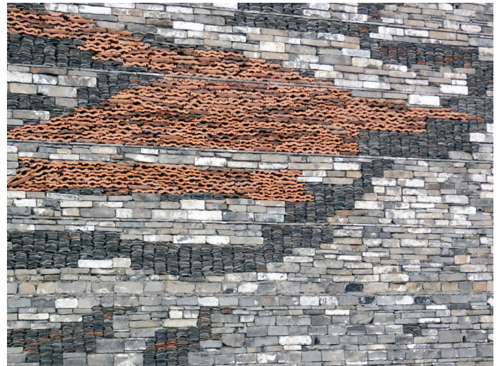
Figure 5. The wapan facade: "a collective work of the craftsmen." Photo credit: Marco Capitanio
